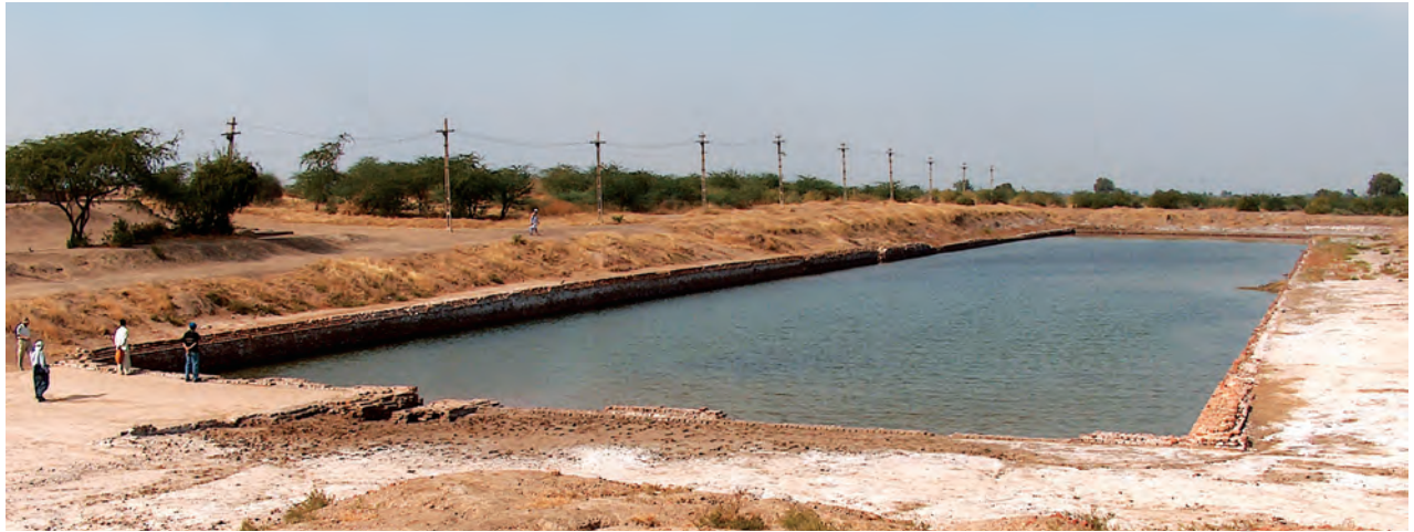
Fig. 6.12. The huge dockyard at Lothal
