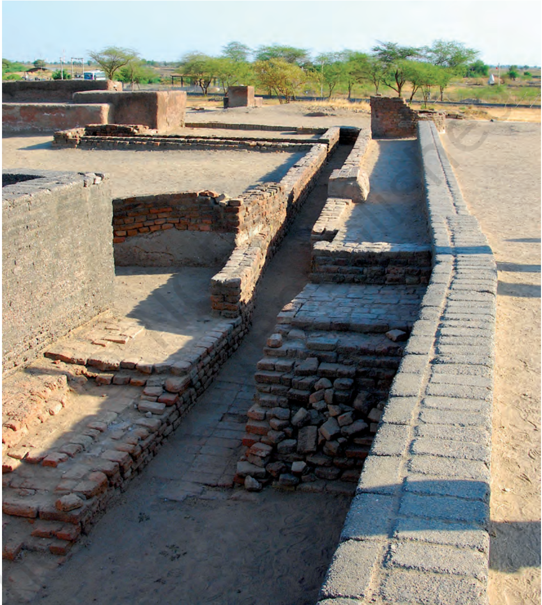
Fig. 6.7. Drainage system at Lothal (Gujarat)
