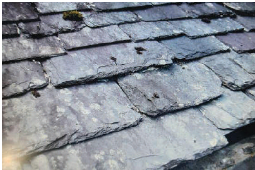
Fig. 11.6: Rocks used for roofing
