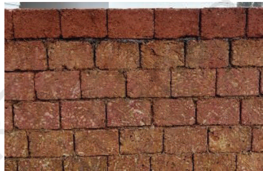
Fig. 11.7: Laterite rocks used as bricks
