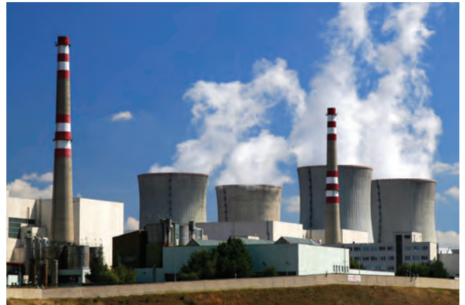
Figure 9.17 : An Atomic Power Generation Plant
