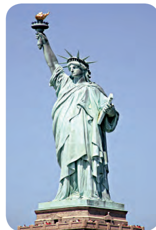
The copper clad statue of Liberty made 300 years ago has turned green.
